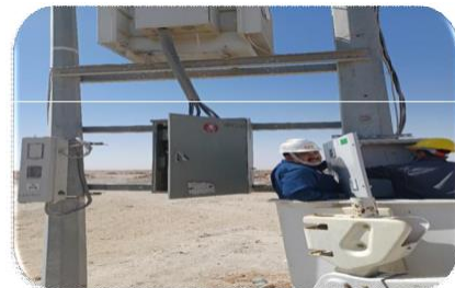
Fig. 10. Installing of feeder monitoring panel
