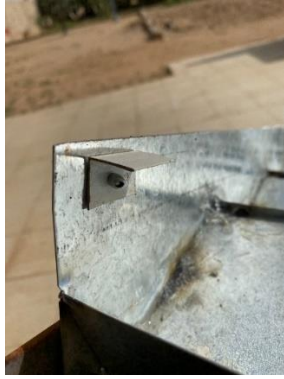
(a) The installation of aluminum stands
