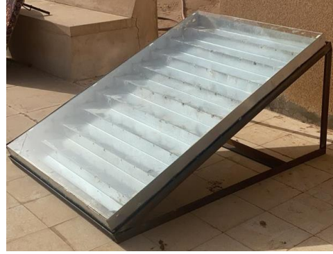
(b) The assembly of the glass cover (with a thickness of 6 mm) on top of the basin
